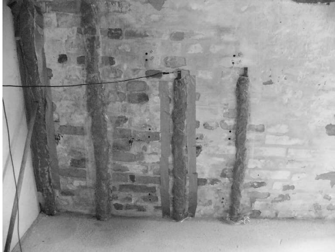
Figure 3: Two sets of electrodes of the pilot plant (first and second set)
